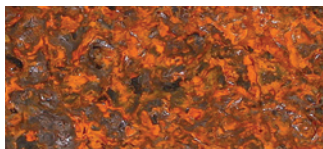
Without corrosion protection treatment
